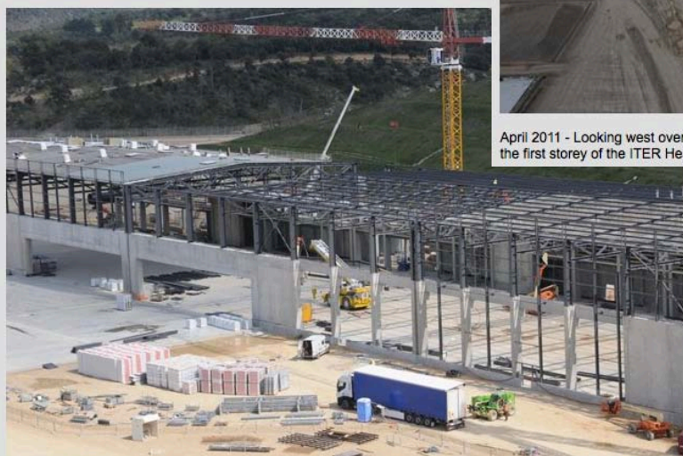
The Poloidal Field Coil Winding Facility is the first building to go up on the ITER platform. 257 m long, 49 m wide and 17 m high, construction will be completed in November 2011. Photo: Spie Batignolles/Altivue
