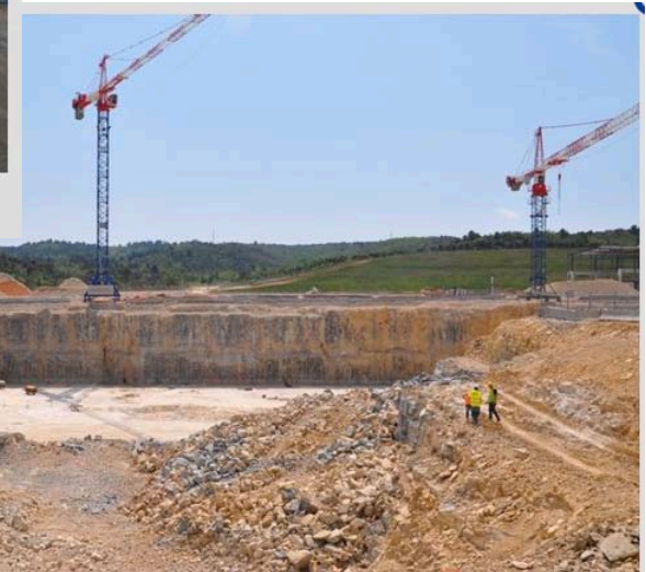
210,000 cubic metres of rock were removed during construction of the Tokamak Complex Seismic Isolation Pit. The Seismic Pit—17 m deep, 120 m long and 90 m—will house the anti-seismic foundations of the future Tokamak Complex. Tower cranes have been positioned at the four corners of the Pit to prepare for the next stage of works: concrete pouring. Photo: ITER Organization (April 2011)
