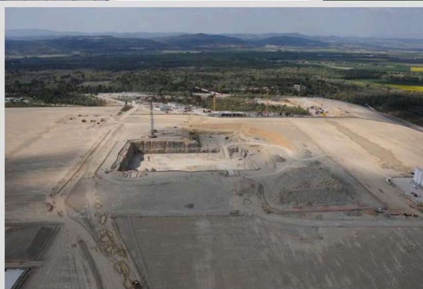
April 2011 - Looking west over the ITER site. Excavation works for the future Tokamak Complex are visible, as well as the first storey of the ITER Headquarters Building in the background. Photo: Altivue
